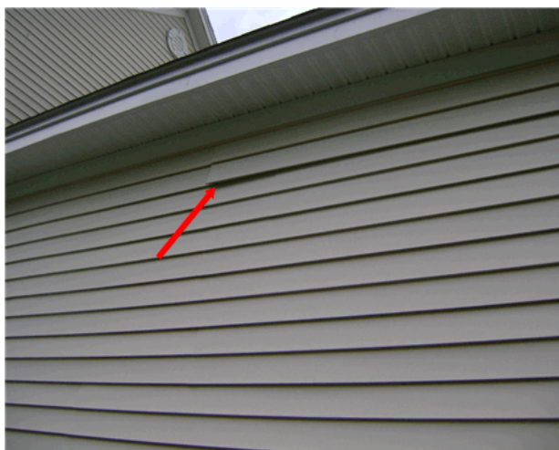
More falling siding
