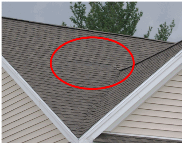
Missing Shingle on roof
