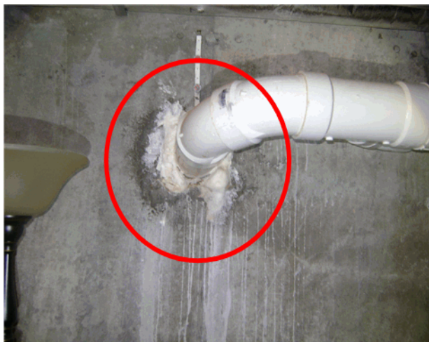
spray foam around drain line
