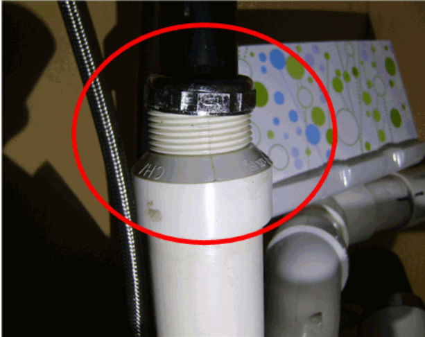
Cross threaded fitting at 1st floor bathroom sink
