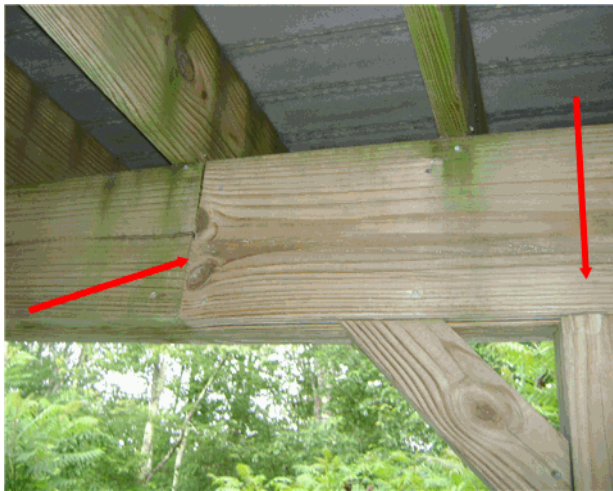
Seams in carriers should fall on a post
