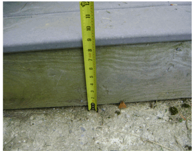
First step on deck stairs is too tall. Maximum of 7 3/4 inches is the standard.
