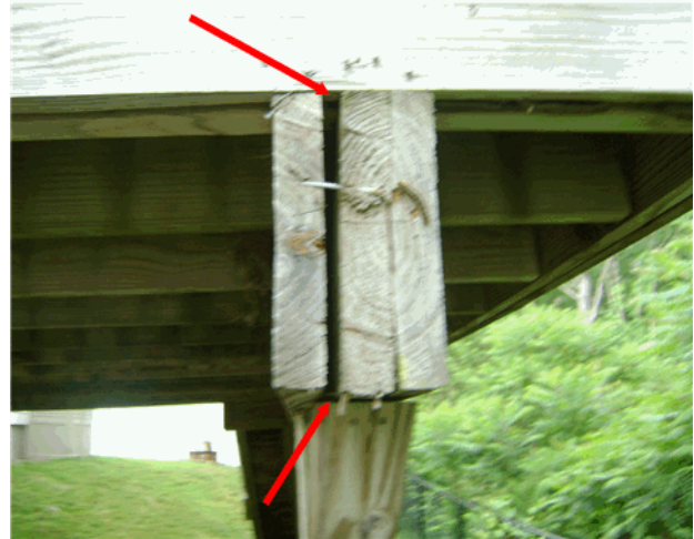
Gap in carrier for deck due to lack of fasteners
