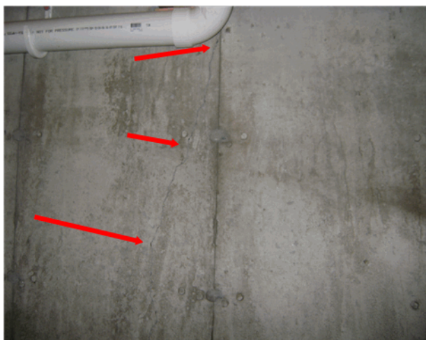
Crack in foundation
