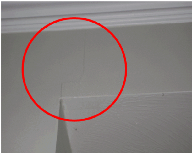
Typical stress crack in master bedroom
