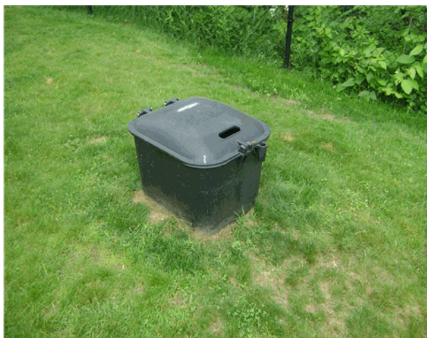
Underground propane tank
