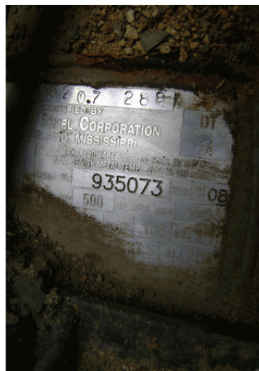
Propane tank info plate
