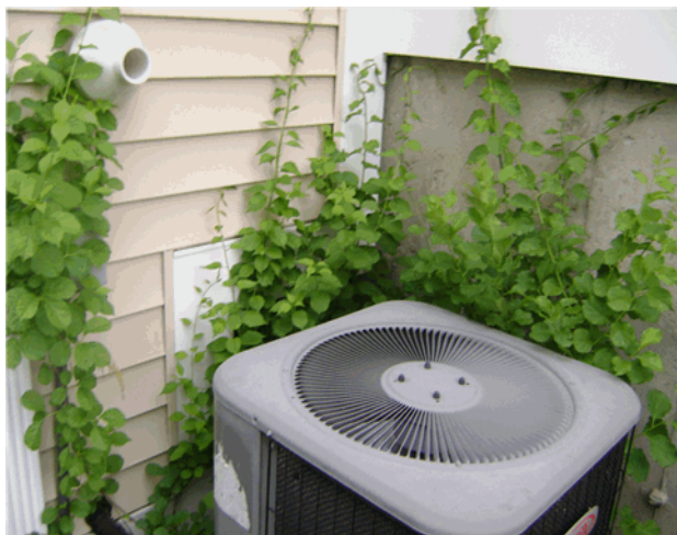
Dense veggitation around condenser
