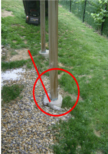
Twisted post due to being undersized
