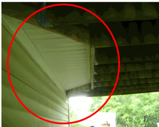
It is not recommended to attach a deck to a bumpout
