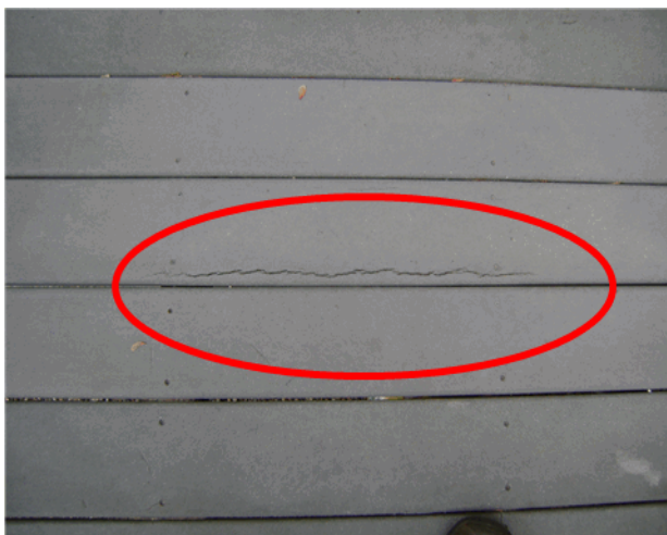
Decking was cracking around screws and in random locations
