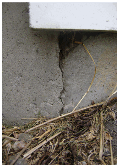
Large crack below garage entry door
