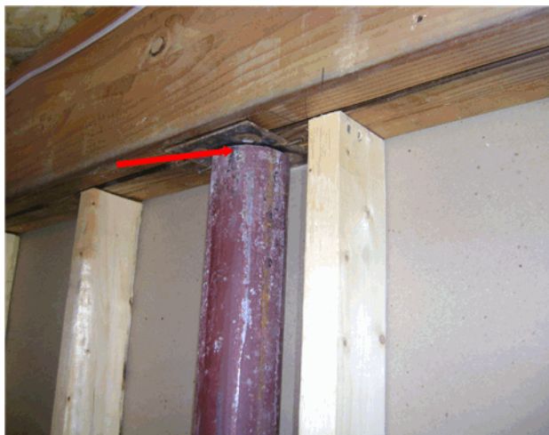
Loose post in basement
