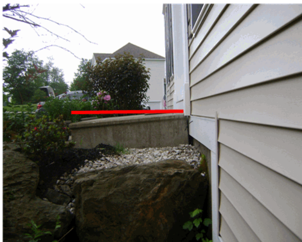
Tilted front steps
