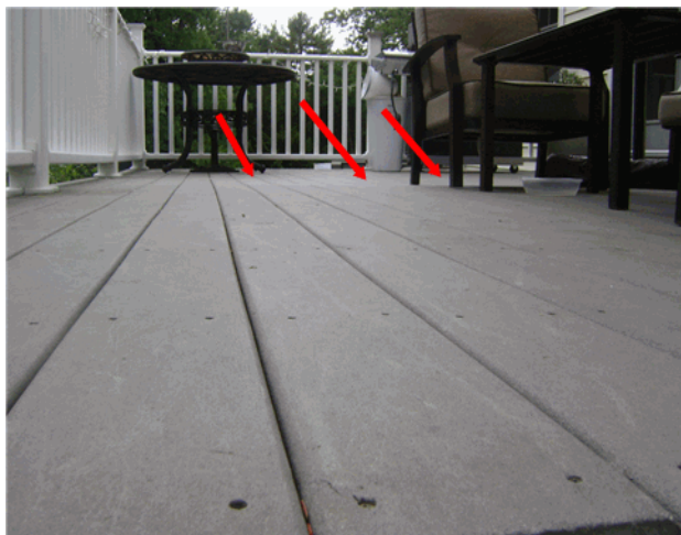
Sag in deck
