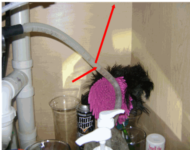
Should be connected making a high loop
