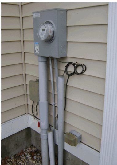
Electrical service and meter
