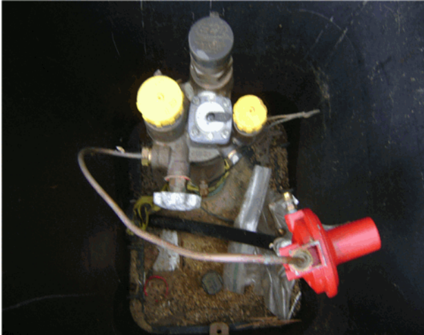
Gas shut off at the propane tank
