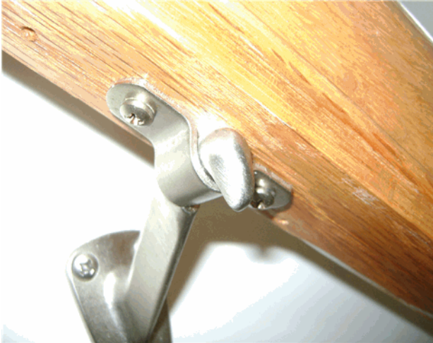
Loose handrail connection at second floor stairway
